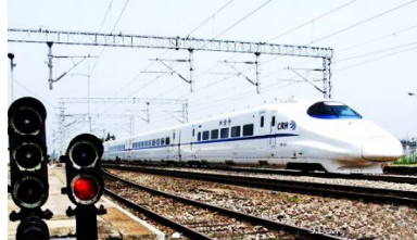
Fig. 1 High-speed railway in operation
